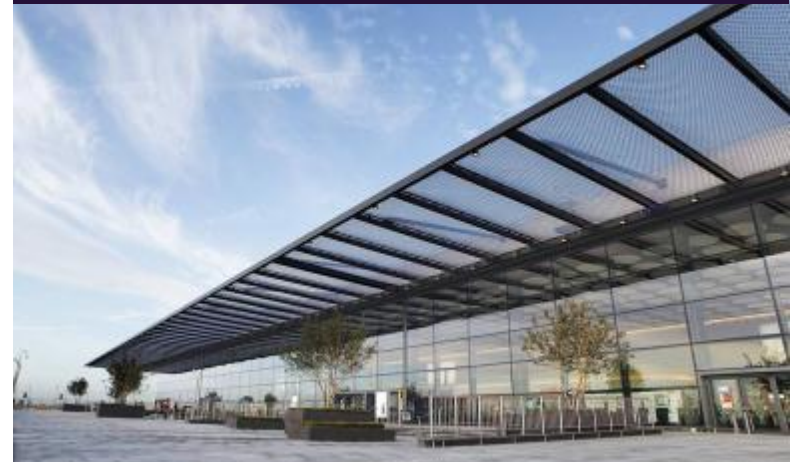
T4: £350m investment in upgrading the terminal since 2007
